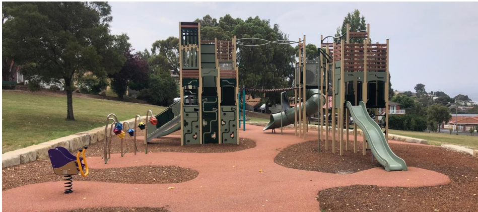
14. Barossa Road Reserve, Glenorchy. Completion Date (July 2024)
