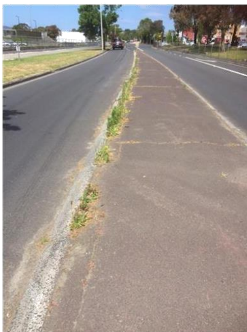
King George V Avenue Northgate Carpark entrance
