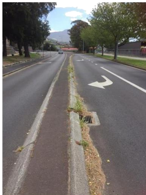
King George V Avenue Northgate Carpark entrance
