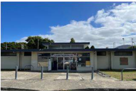
Image 10: Aged ingress point
