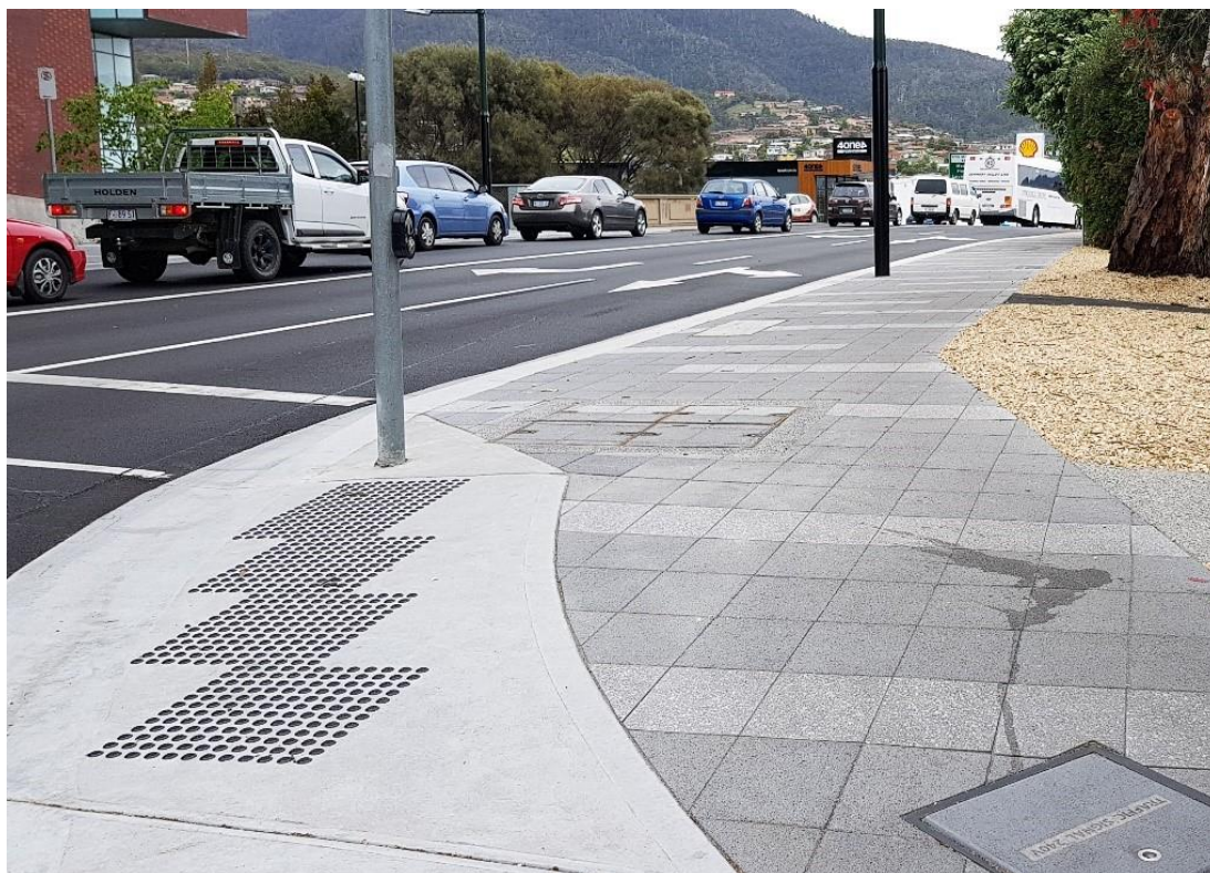
Figure 3 Stage 2 footpath on Main Rd opposite ICC
