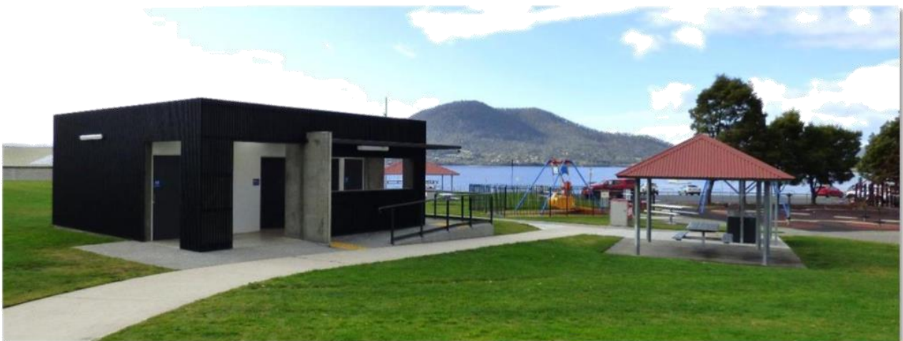
Below: Montrose Bay Foreshore toilet block
