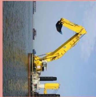
1.2 Dredging to remove silt of marina and allow access to larger boats
