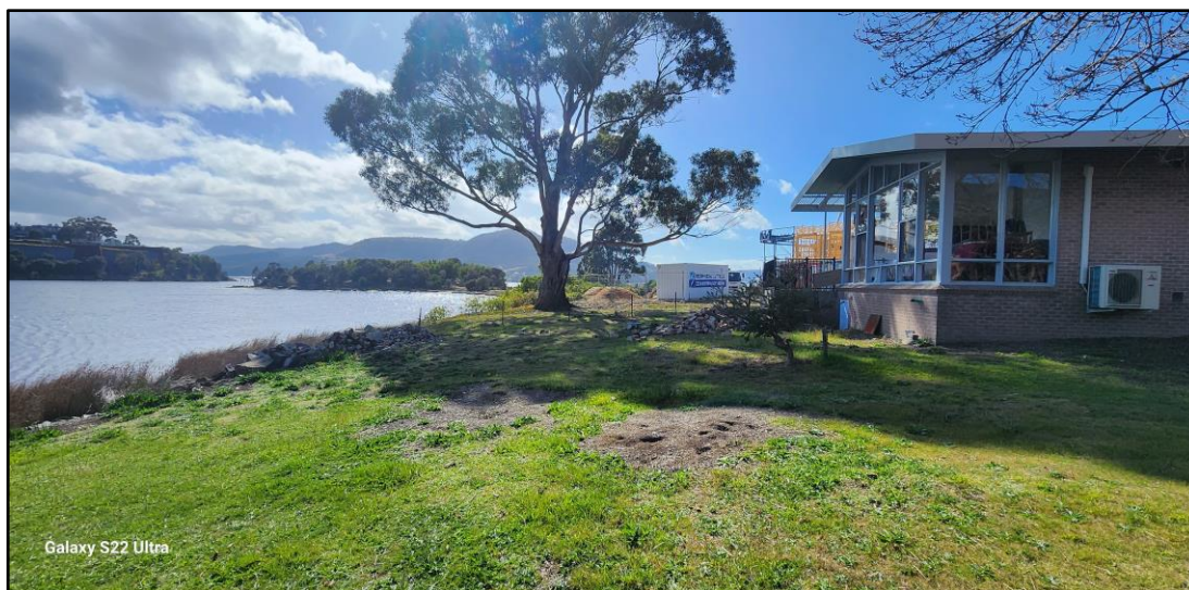
Figure.13: Showing the private open space at rear of the property 7 Strathaven Drive, Rosetta
