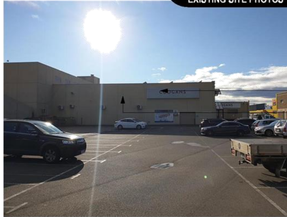
EXISTING CARPARK FROM CHARLES STREET
