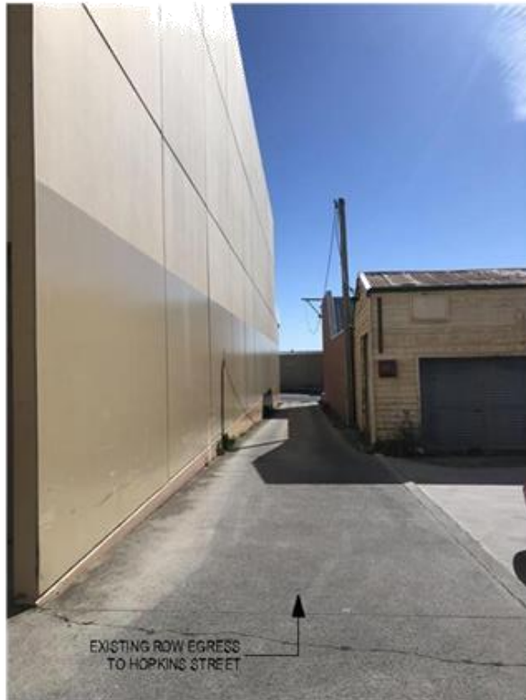
EXISTING ROW ACCESS FROM HOPKINS STREET
