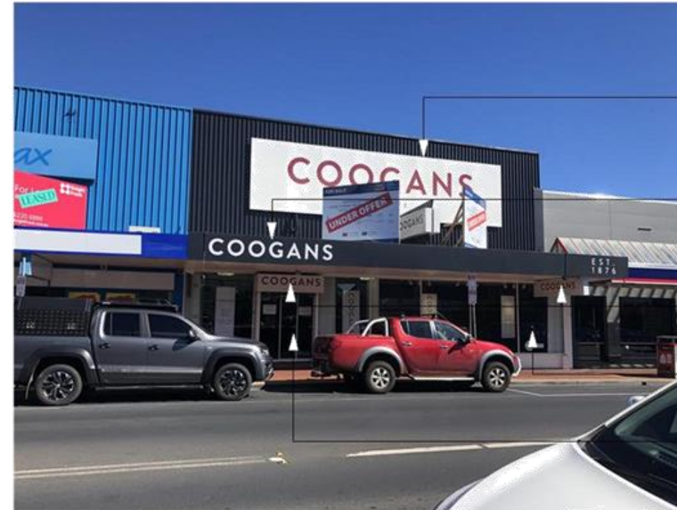
EXISTING 80-82 MAIN ROAD VIEW
