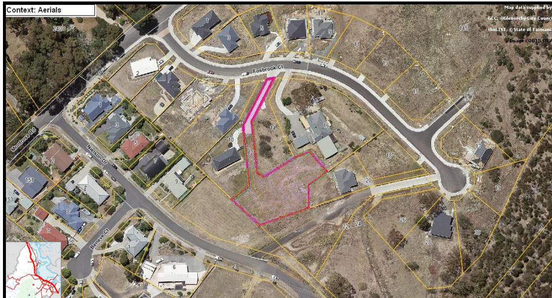
Figure 1. An aerial snapshot of the site and surrounds, Council record, Exponare.
