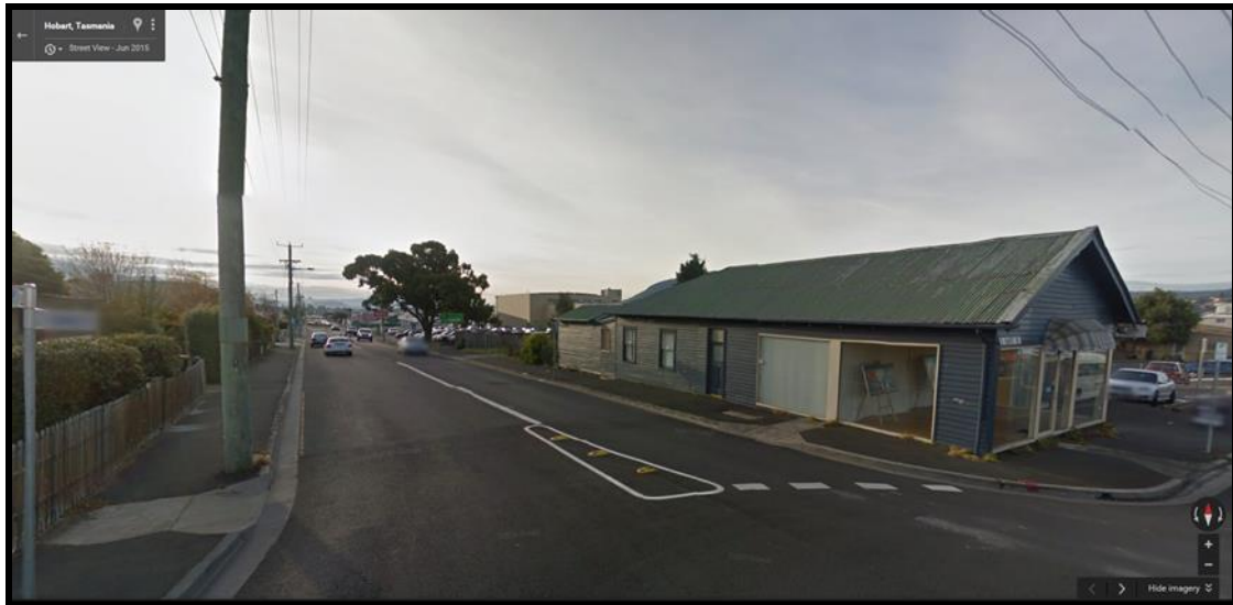
Figure 2. A snapshot from Street view, showing the existing building with direct access to Albert Road and Charles Street.
