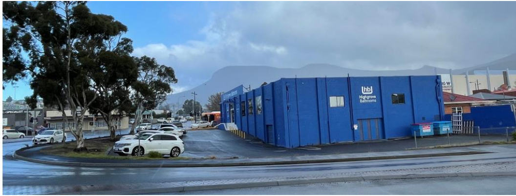
Figure 8 – 345 Main Road, Glenorchy looking south.
