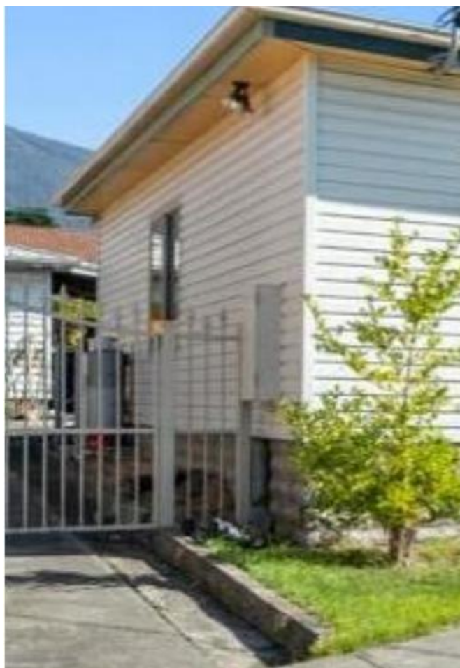
Figure 3. A view of the existing habitable room window on the north-eastern elevation of the existing dwelling that is to be fitted with translucent glazing to a height of 1.7 m above ground level and is within 1m of the proposed shared driveway.
