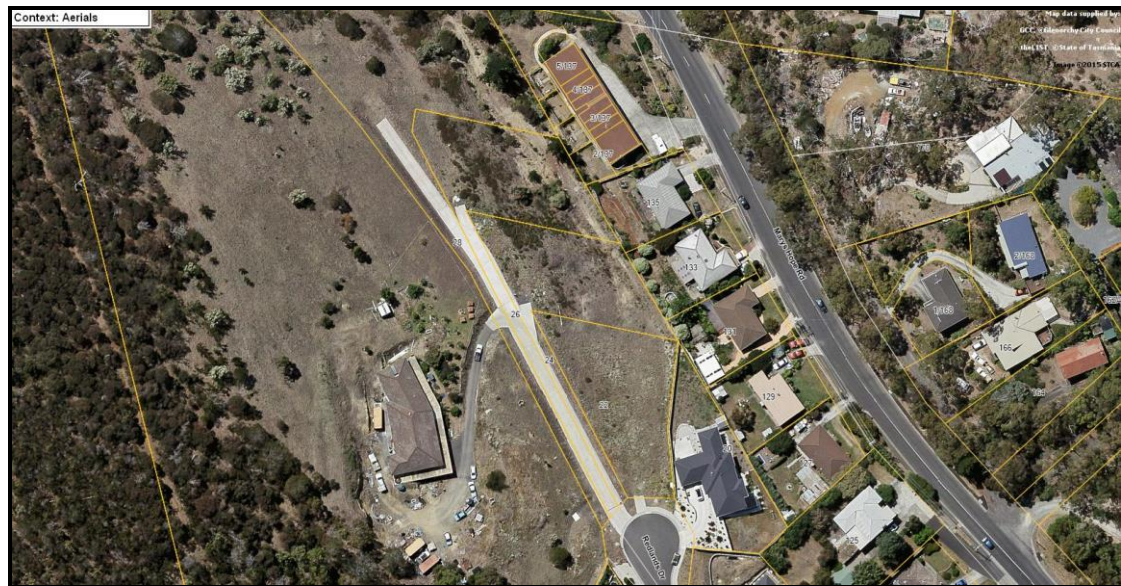
Figure 2: Aerial photograph of 26 Redlands Drive, Rosetta.
