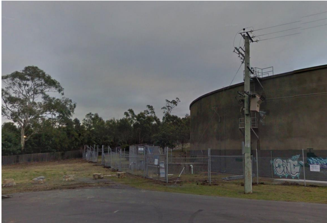
Figure 8: View of the reservoir and TasNetworks infrastructure.
