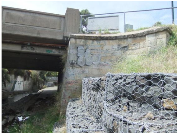
O'Brien's Bridge sandstone wing wall and abutment south-east corner. (Source: GCC photo)
