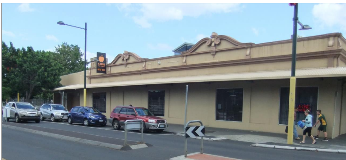
The façade of Hickman's Store remains clearly discernible in the present despite the loss of detail.
