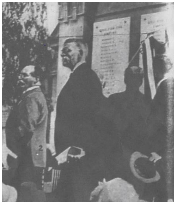
1922 photo showing the panels in their original position at the opening of the Soldier's Memorial outside the old Council Chambers. (Source: Tasmanian Mail in GCC collection)
