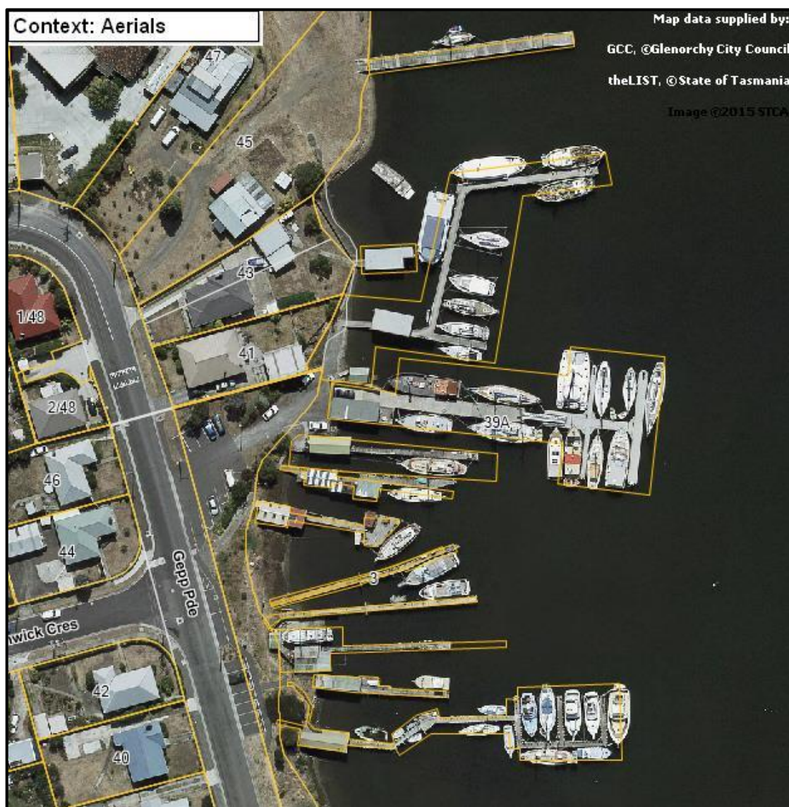
Figure 3: Aerial photo of the site at Gepp Parade and 1 Gepp Parade, Derwent Park.
