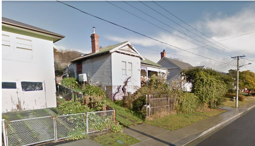
Figure 1. The street view of the dwelling to be demolished.
