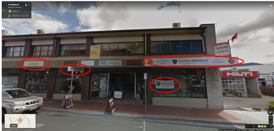
Figure 8. Photograph of the eastern end of the Hopkins Street façade of the building, showing existing signage for Tasmanian Numismatics and Darcy's Café (circled in red) – Google Street view 2016
