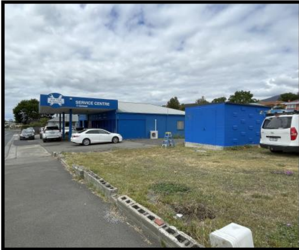
Figure 2 – View to existing buildings on the land from Main Road
