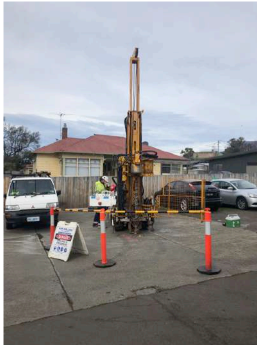
Drilling of MW02
