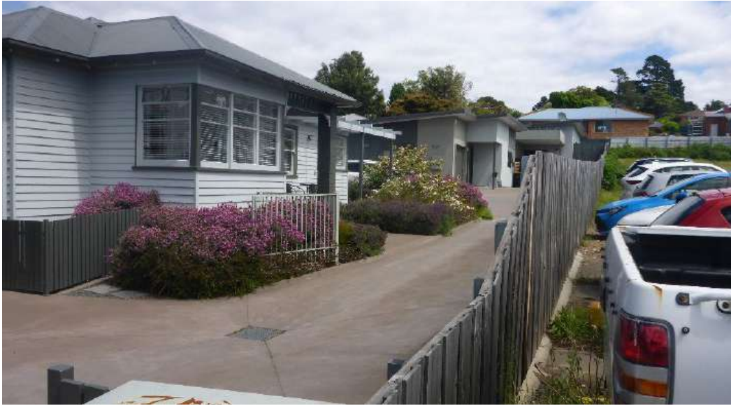
Photo 5: interface of the subject site with Nos. 1, 2 and 3/6 Main Road
