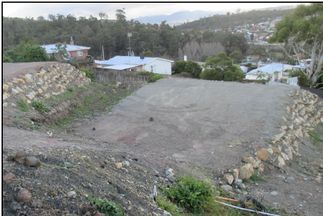
Figure 3. A view of lot 12, the subject site, showing the buildable area with embankment bordering the site to the east, north and west.
