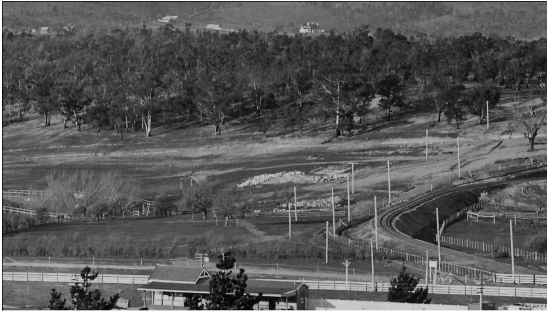
Figure 10 - Enlargement from a panoramic view circa 1920 showing the neck of land leading to Triffitt's (now Dogshear) Point corresponding to the Cadbury rail spur, and which was to become the site of the Claremont Primary School. The levelled (and now archaeological) remnants of 'Ashburton' on the low hillside are clearly visible, just to the right of the centre in the photograph. (Source: Crop and enlargement of a photograph presented to GCC by Mrs M Smith)
