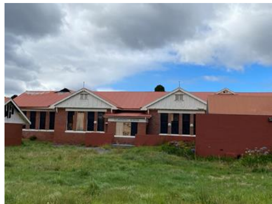
2a. Front view of part of the main school building.
