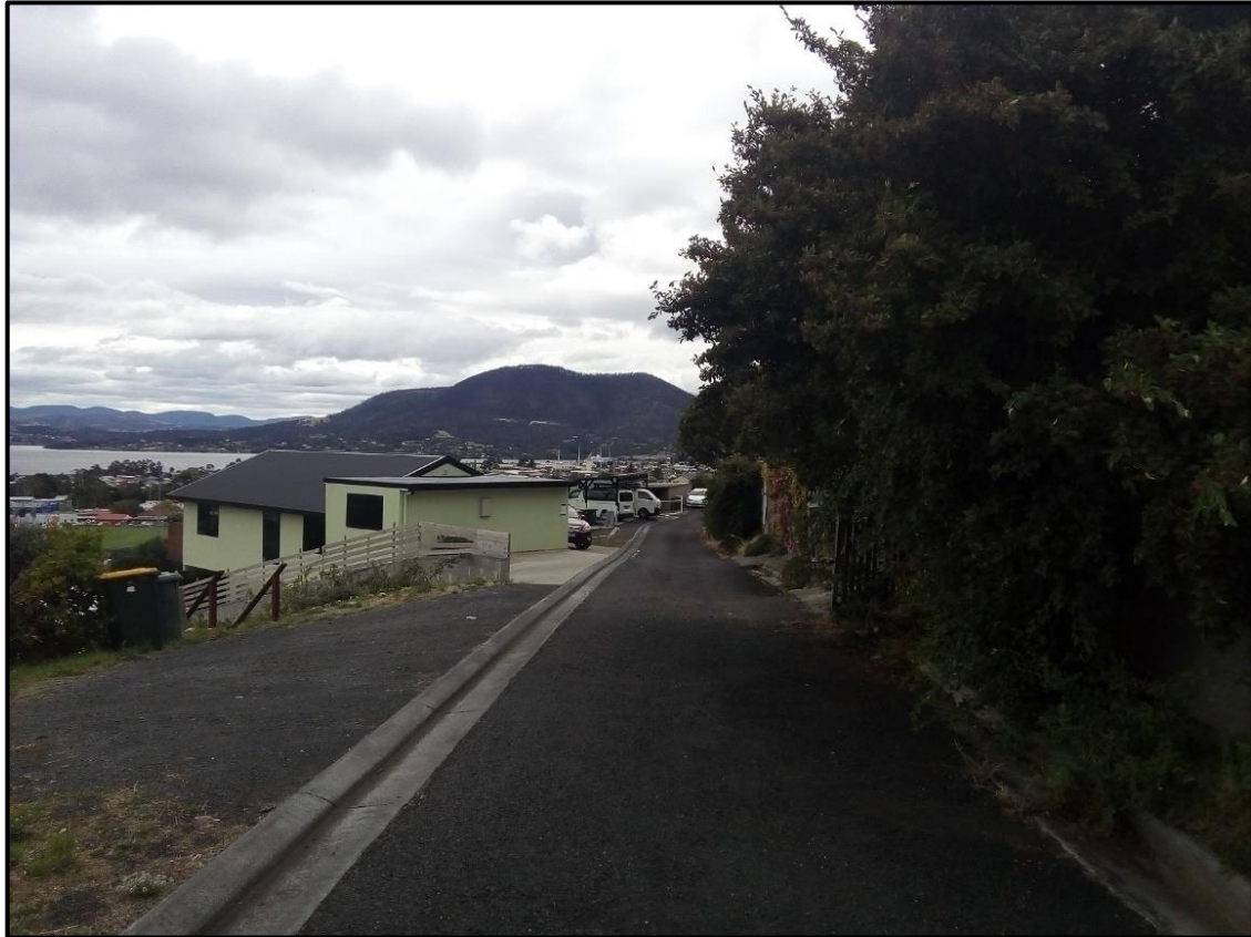
Figure 3 :Unnamed service road (2/10 Bowden St. in mid-distance)
