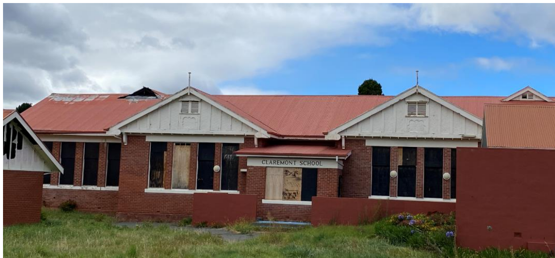
Figure 4 – Front view of the main 1924, 1938, 1941 school building partly obscured by intrusive structures, boarded up, neglected, vandalised and partially damaged by fire but retaining its Inter-War architectural character and pre-eminence in the former school buildings complex (Source: GCC image, 26/2/2021)
