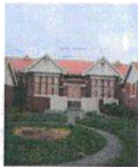
Claremont Primary School Block A DPIPWE May 2012
