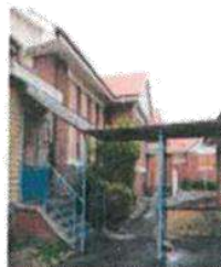
Block A (centre), Block D (left), Block C (right) DPIPWE May 2012
