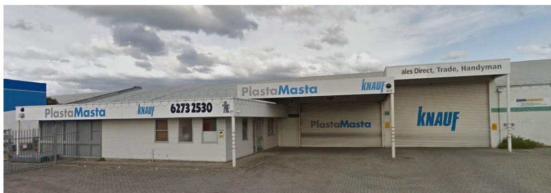
Figure 4. View indicating existing Awning Fascia signage.
