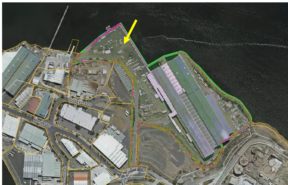
Figure 2 - An aerial view of the subject site (the arrow indicates the location of the proposed extension/stage 2 development) and surrounds.
