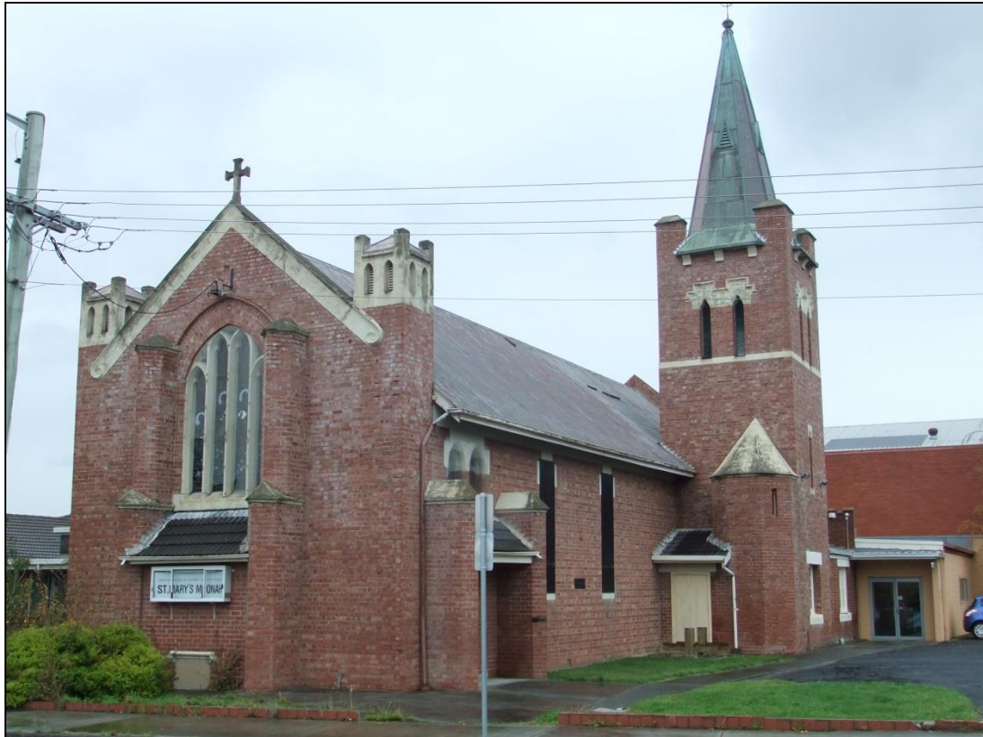
General view of St Mary's Anglican Church from Springfield Avenue.
