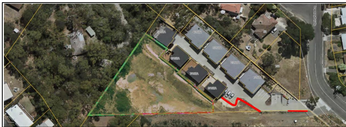
Figure 10: Areas without retaining walls currently
