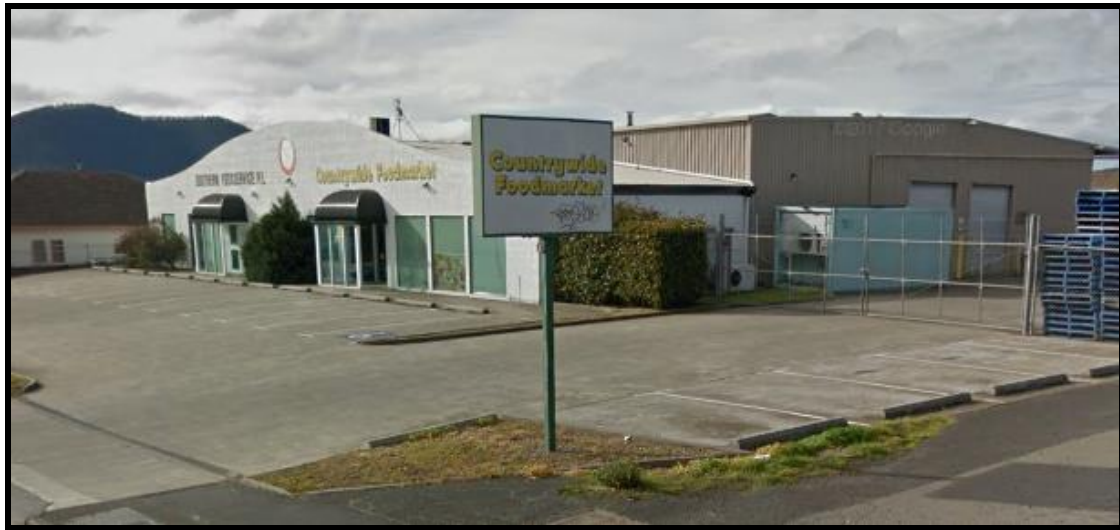
Figure 2. Photograph of the site showing the existing sign – Google Streetview image June 2015
