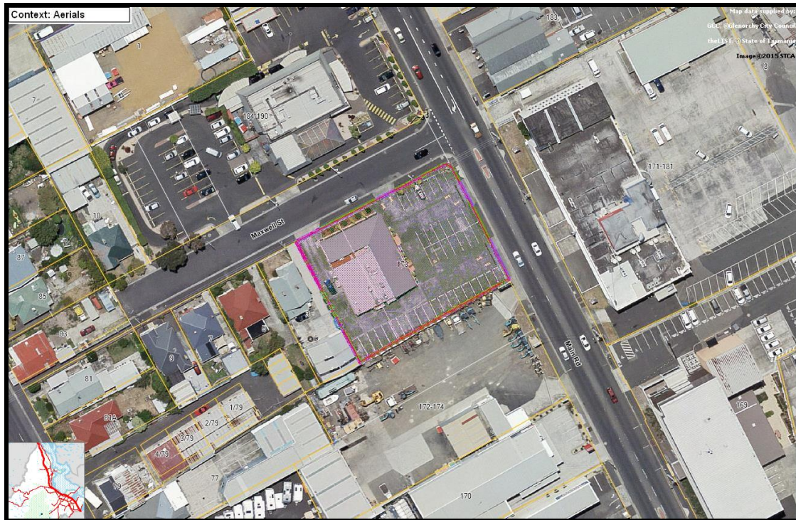
Figure 1. An aerial view of the proposal site, showing the site and surrounds, Council record, Exponare.
