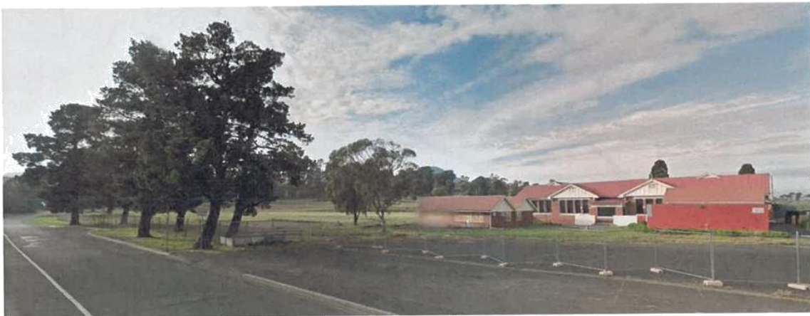
Figure 5 Site image – looking south
