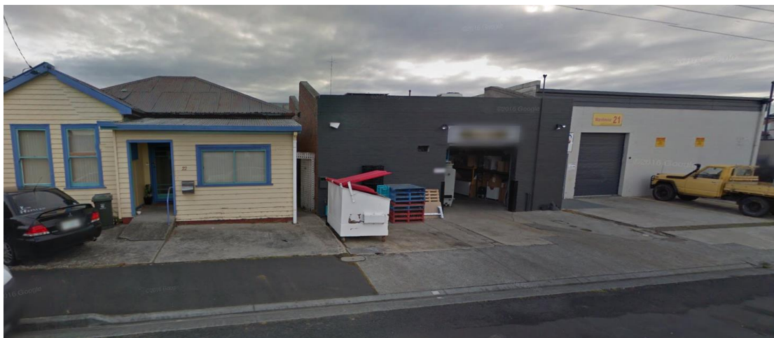
Figure 4. Wide vehicle access traversing 22 Station Street (weatherboard building) and 51-53 Albert Road (dark grey brick building), Google Street View
