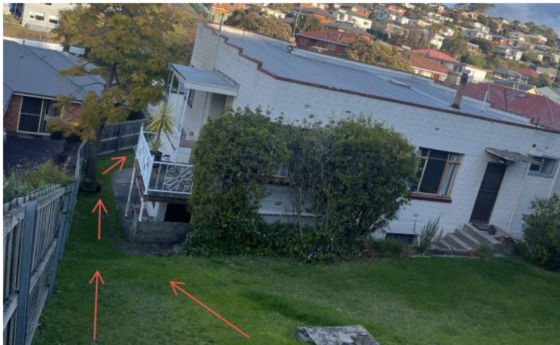
Figure 5 - From rear of 5 Second Avenue looking southeast at rear of 74 Springfield Avenue
