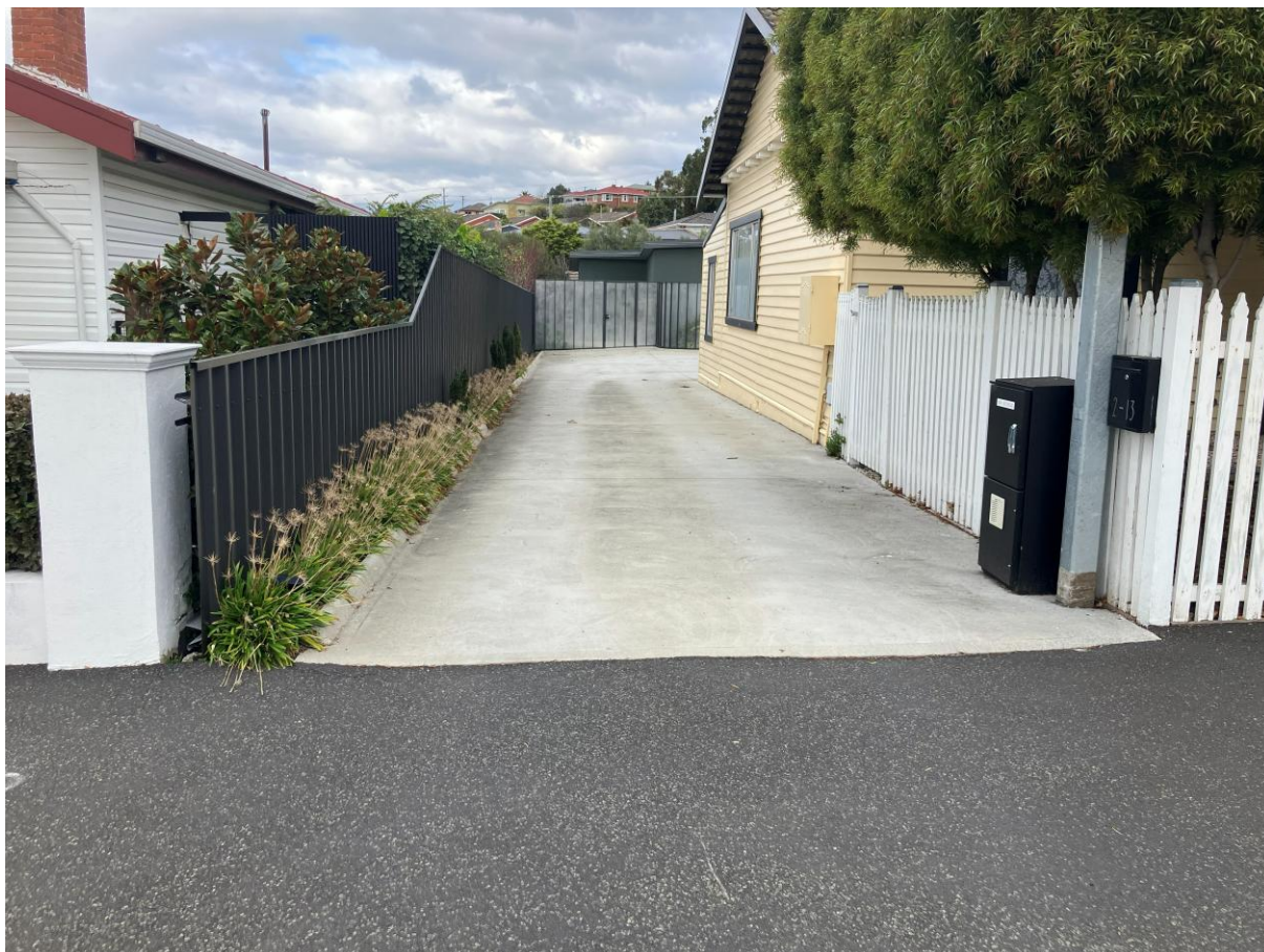
Figure 6: Neighbouring driveway kerb directing overland flow away from the proposed development area.
