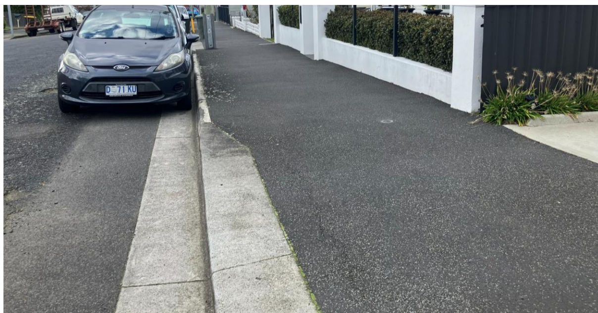
Figure 5: Front of property showing kerb and channel.
