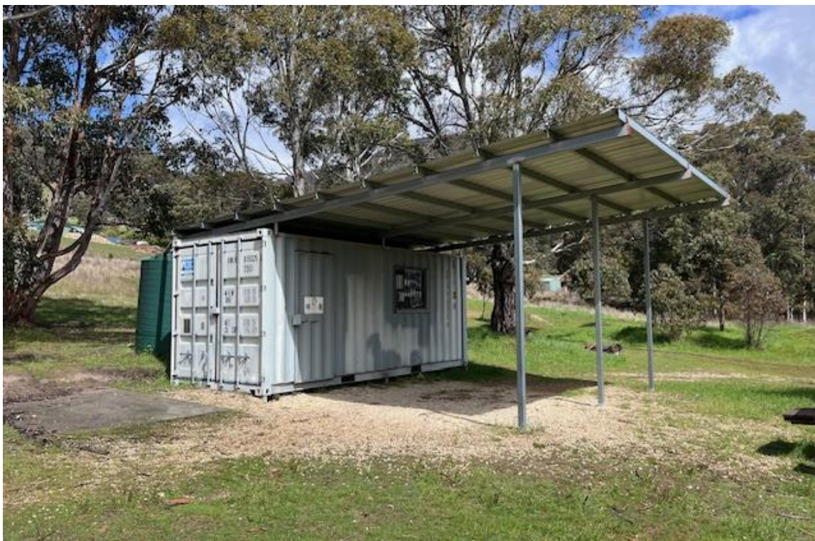
Figure 2 – Existing shipping container and shelter
