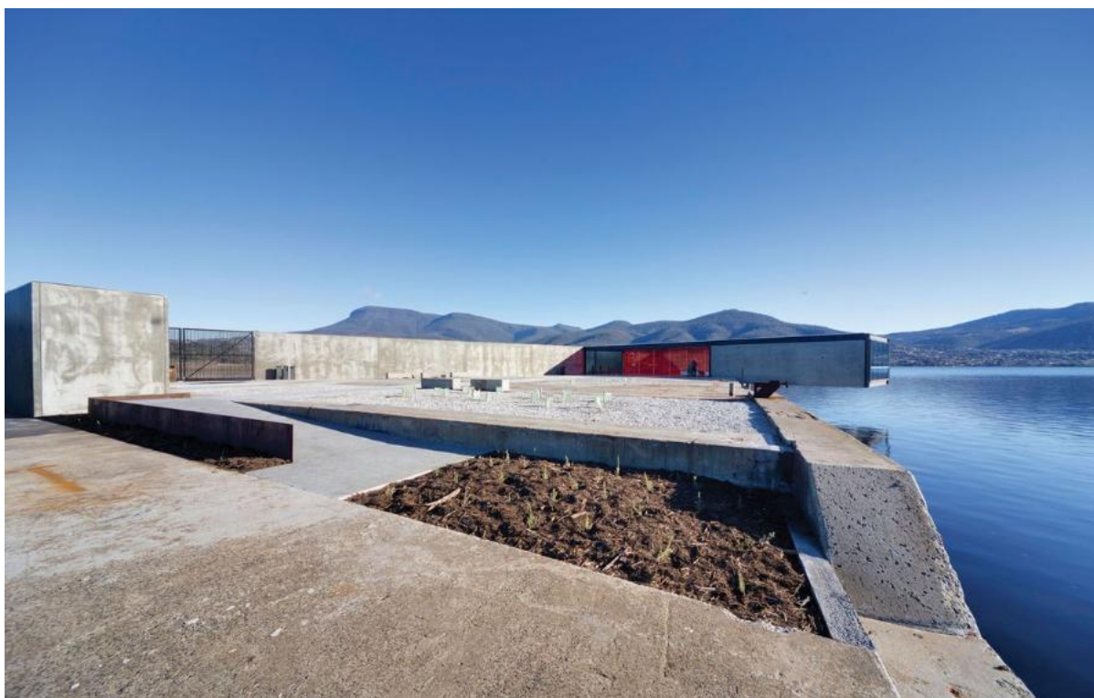
Figure 5: View of point infrastructure with GASP! Pavilion and the toilet block (left in image) and dock (Source: https://architectureau.com/articles/gasp/#img-5 )
