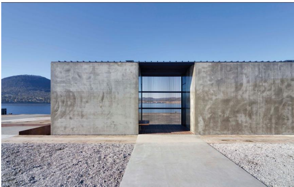
Figure 4: View of existing toilet block, looking east (Source: https://architectureau.com/articles/gasp/#img-5 )
