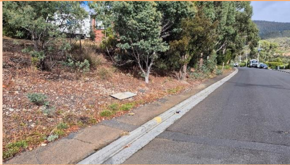
Existing fire plug – Abbotsfield Road
